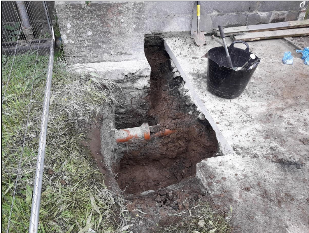
Photograph 7 – Concrete strip initially removed beside contaminated soils (27.07.20)
