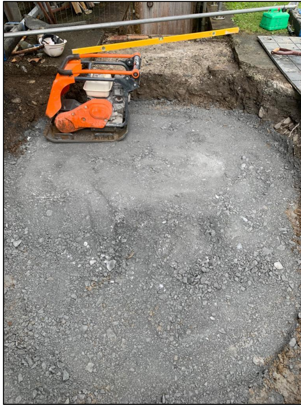
Photograph 16 – Excavation backfilled with MOT compacted in layers (13.08.20)
