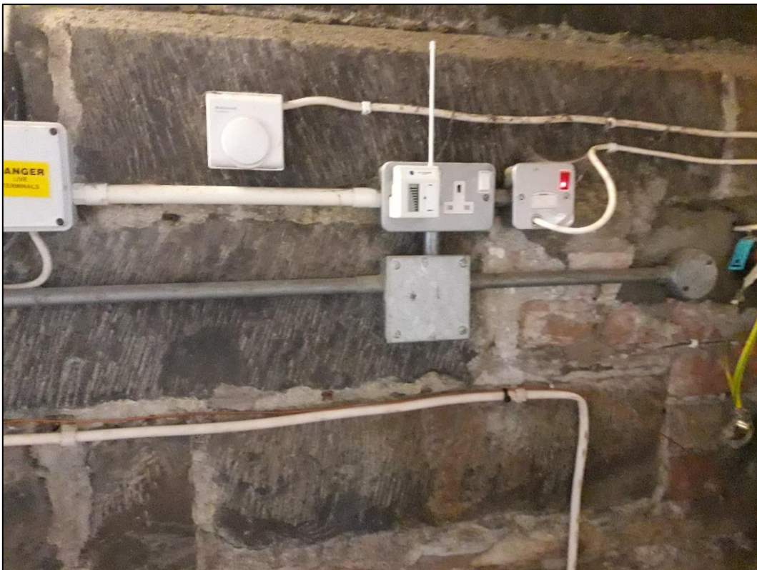
Photograph 25 – Electronic fuel level monitor in the boiler room (01.09.20)
