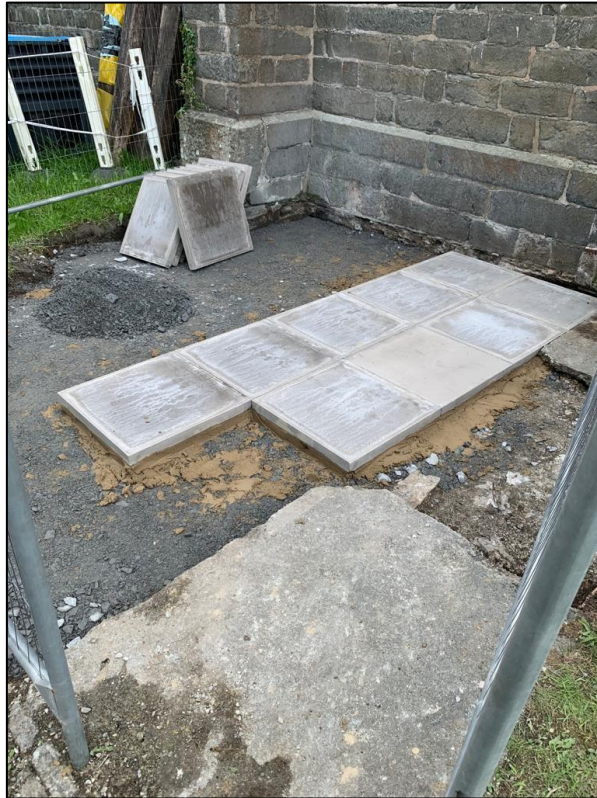
Photograph 18 – Concrete slabs laid onto compacted surface to form OST base (13.08.20)
