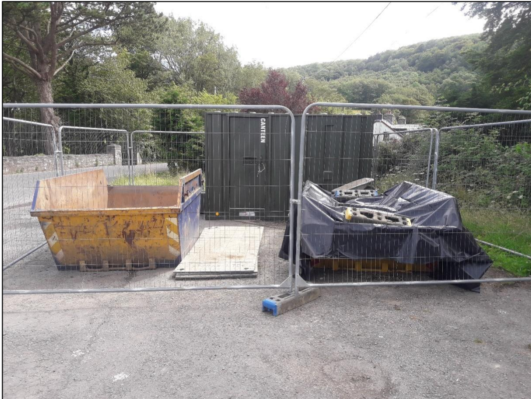
Photograph 13 – Skips and welfare unit in fenced compound in lay-by (30.07.20)
