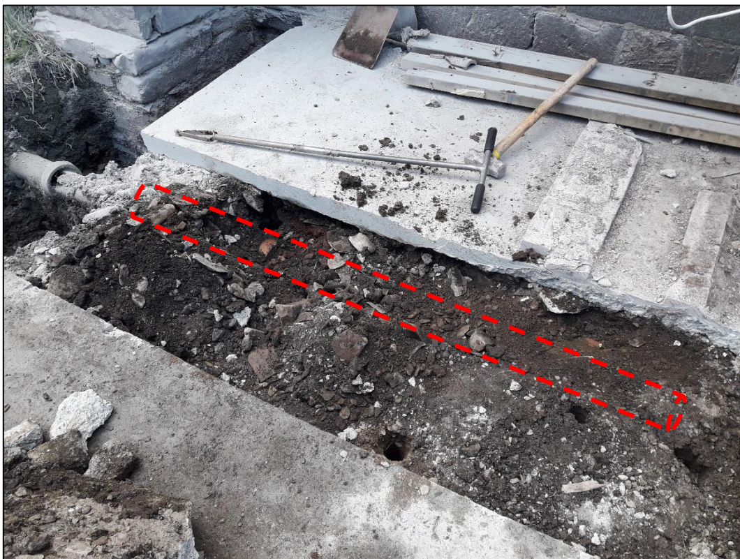
Photograph 10 – Redundant clay pipe unearthed, route highlighted (28.07.20)
