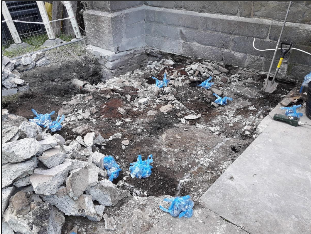
Photograph 13 – Validation (V) samples retrieved from beneath the concrete pad (28.07.20)
