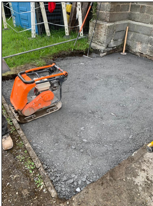
Photograph 17 – Excavation backfilled to ground level (13.08.20)
