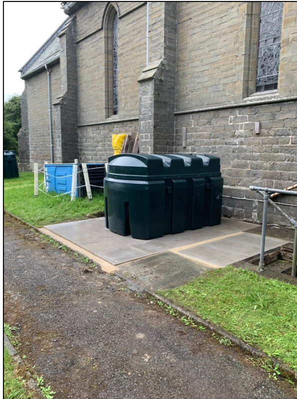
Photograph 20 – OST positioned on concrete slabs (17.08.20)
