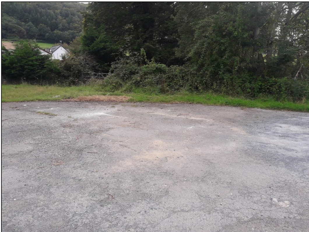
Photograph 27 – Lay-by brushed down and left clean and tidy (01.09.20)
