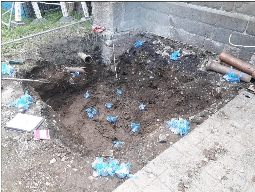
Photograph 14 – Excavation Validation (EV) samples retrieved (30.07.20)
