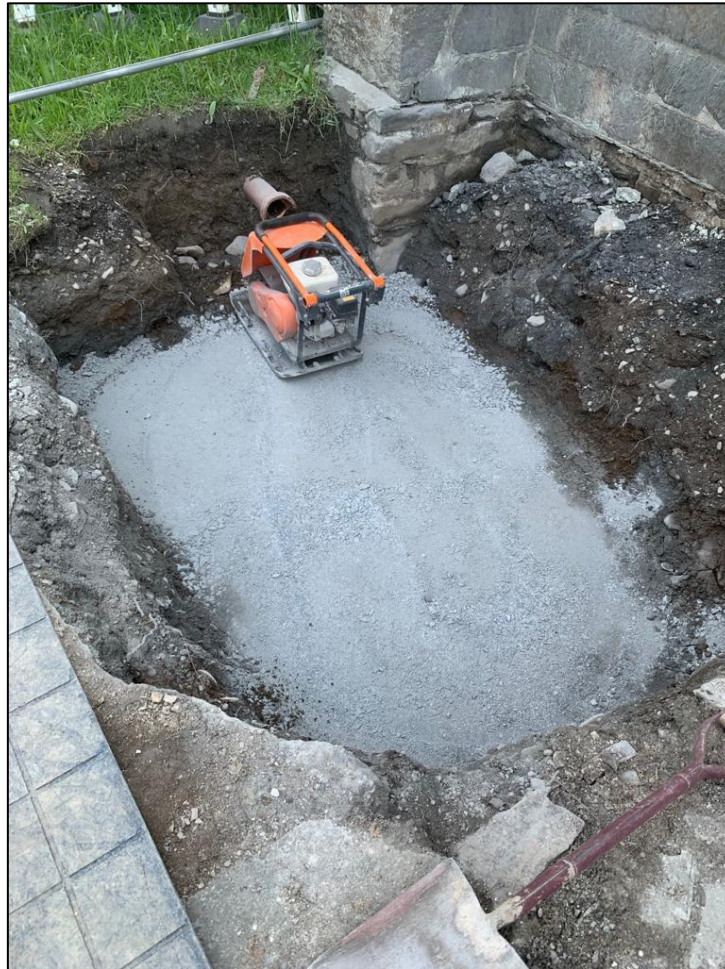
Photograph 15 – Excavation backfilled with MOT compacted in layers (12.08.20)
