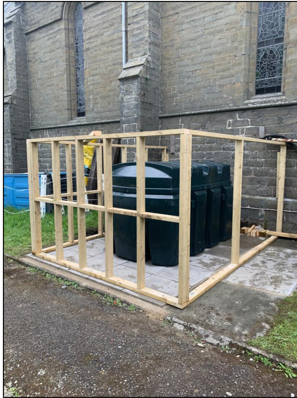
Photograph 22 – Timber frame constructed around the OST (21.08.20)
