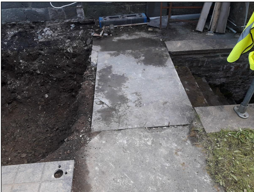
Photograph 12 – The slate slab had to be removed during remediation works (30.07.20)
