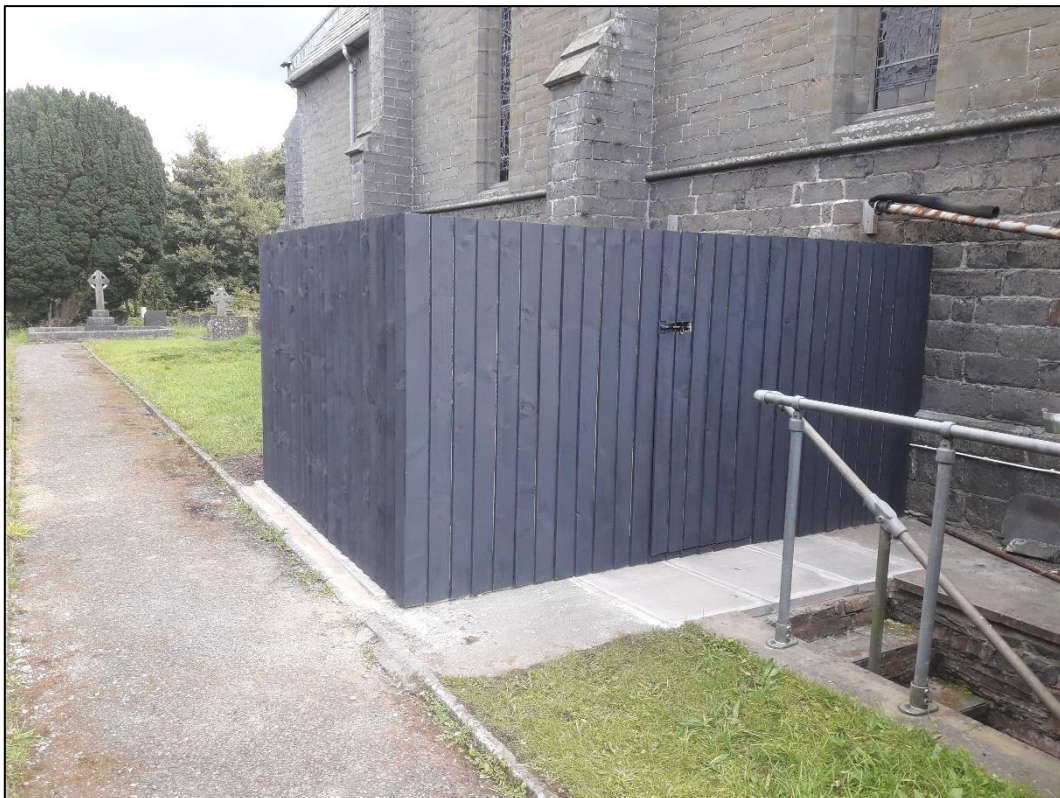
Photograph 23 – Timber surround installed around OST to match previous style (01.09.20)
