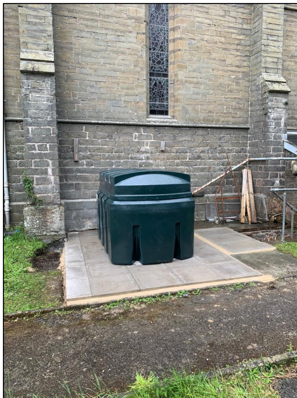
Photograph 19 – Concrete slabs laid to form OST base (17.08.20)
