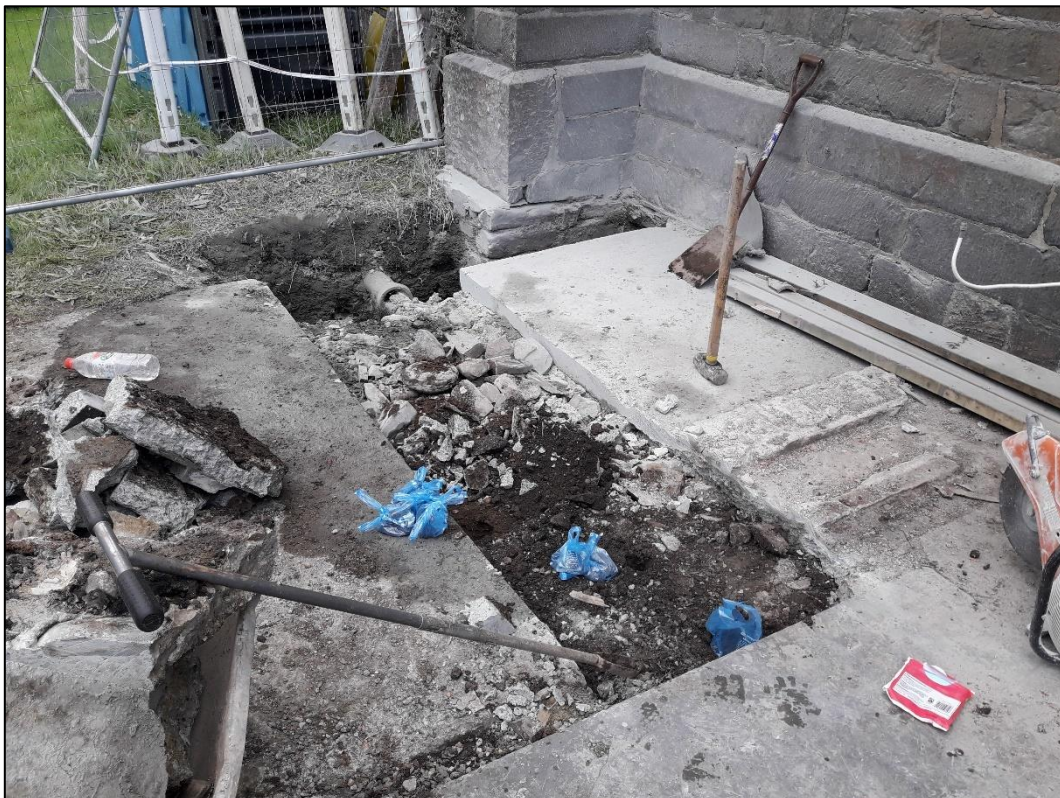
Photograph 8 – Concrete strip broken out, tracking contaminated soils beneath (28.07.20)
